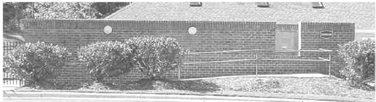
Solid walled enclosure for trash compactor with foundation landscaping
