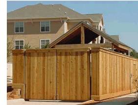
Gated Access to Trash Enclosure
