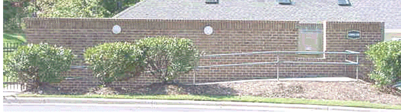
Solid Walled Enclosure for Trash Compactor with Foundation Landscaping
