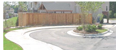
Vehicular Pull-Off at Trash Enclosure
