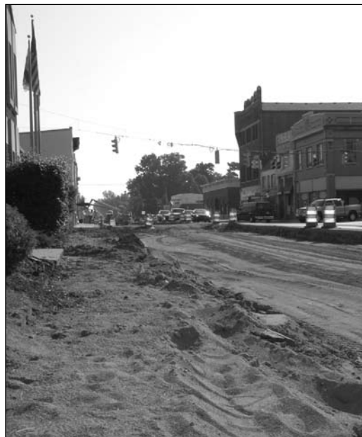
Construction on the Town Center Streetscape Project.
